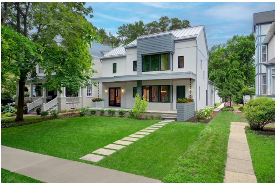
Passive House, 1210 Maple Ave. Credit: Nate Kipnis
