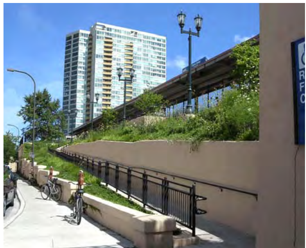
Metra Station ADA Ramps
