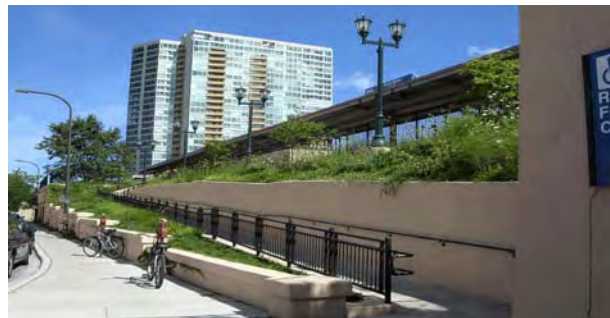
Handicapped Access Ramp on Maple Avenue
