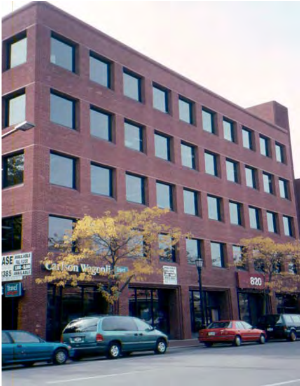
New 820 Davis Street Building
