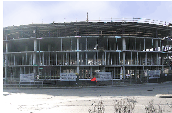
Grand Bend @ Green Bay Under Construction
