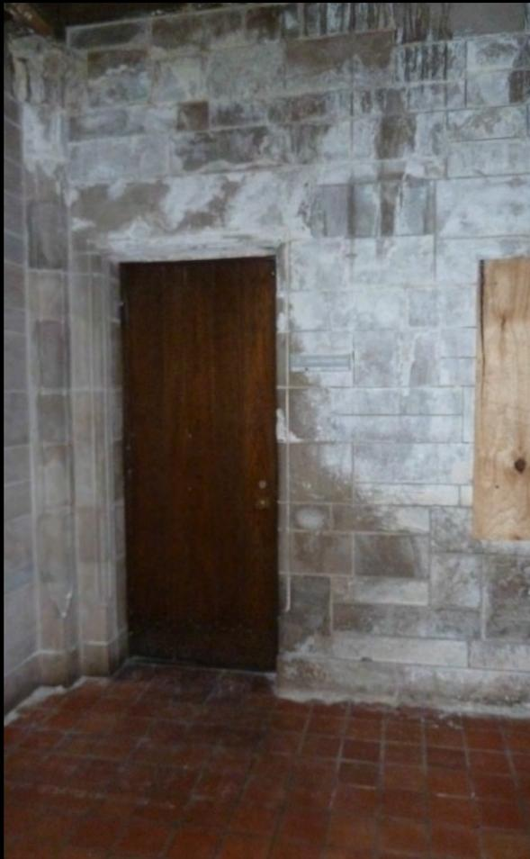
Damaged condition of stone walls at corridor.
