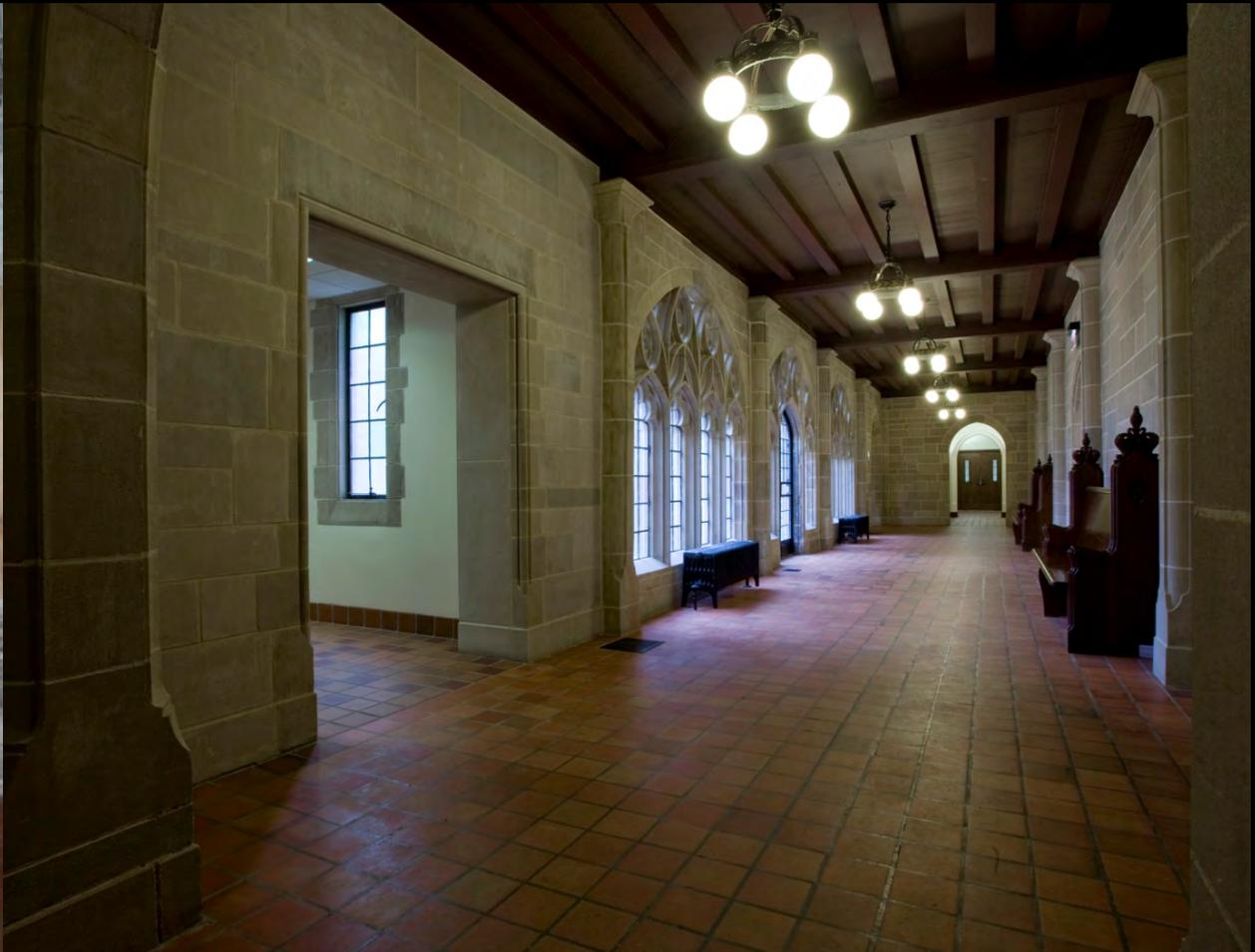
Main corridor with restored finishes and light fixtures and new opening at left with reused existing carved limestone jambs
